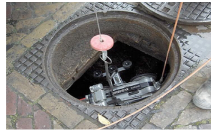
Figure 5 – Example sewerage inspection
