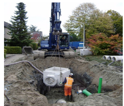
Figure 6 – Example sewerage inspection
